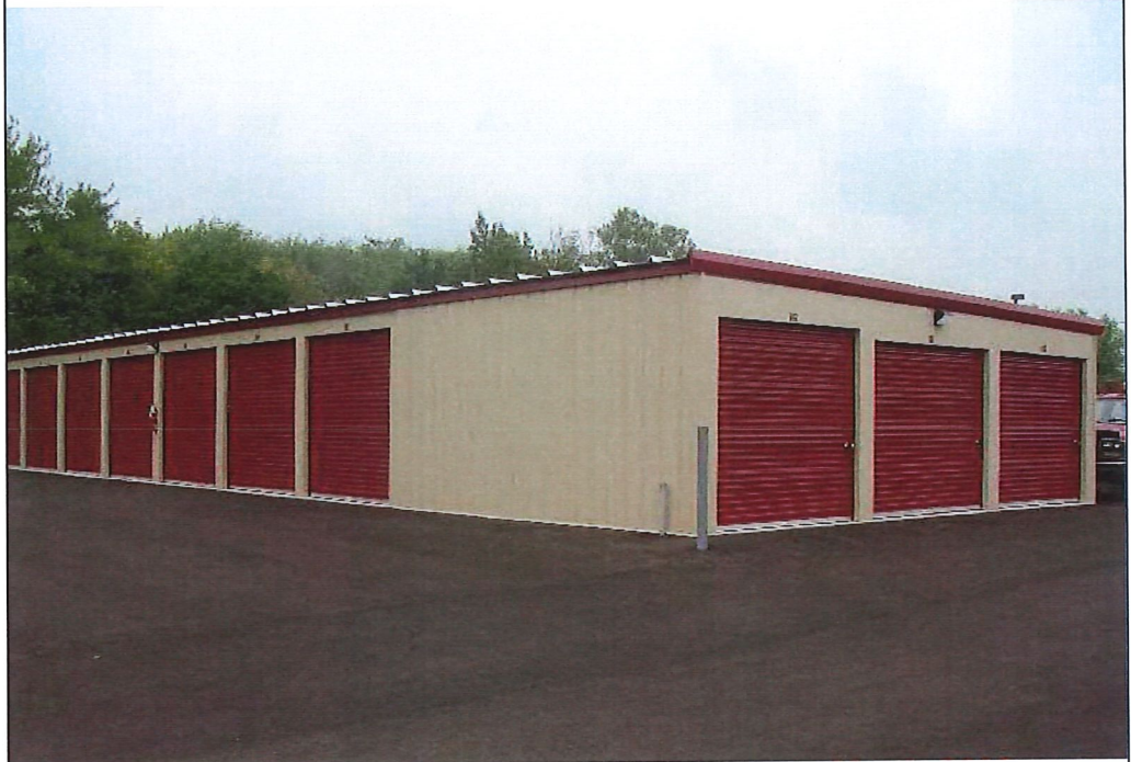
A lean-to building with Garnet doors on the high and low sides.
