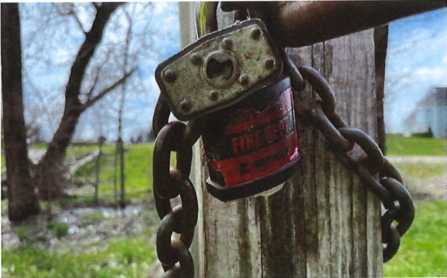
Figure 3 – Installed Knox Box
