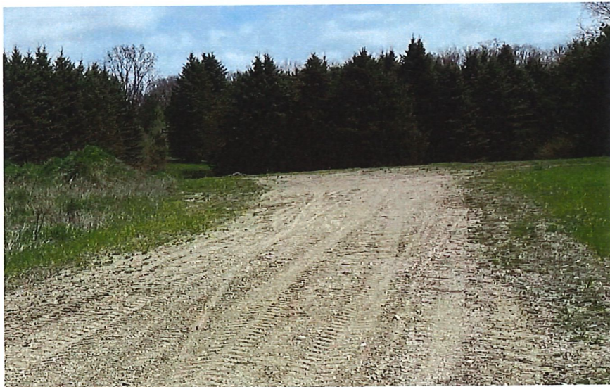
Figure 5 - Construction Debris No Longer Present in May 2022
