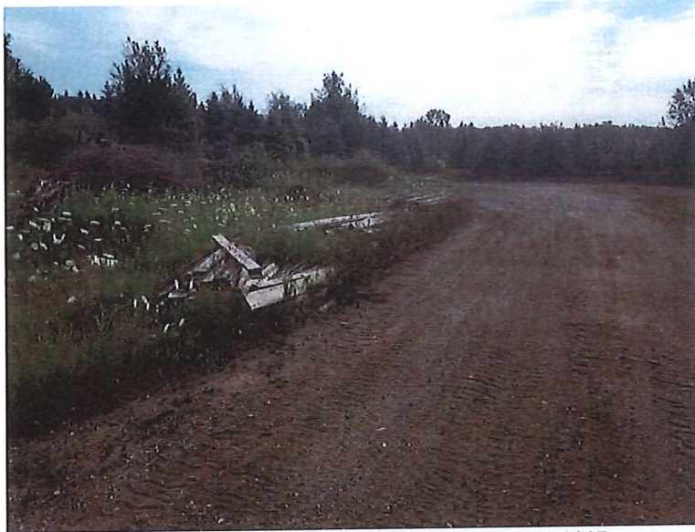
Figure 4 - Construction Debris Noted in August 2017
