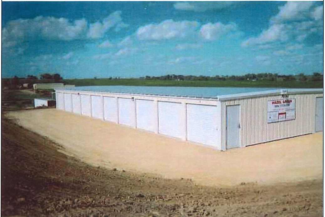
Cream Beige building with Iced White doors and trim. Note: The swing door on the end wall is for ADA compliance. (American Disability Act)
